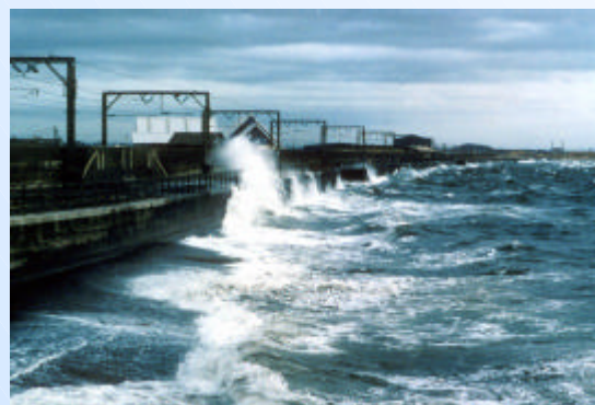
Figure 2: Overtopping of seawall onto main railway - Saltcoats, Scotland (photo: Alan Brampton)
