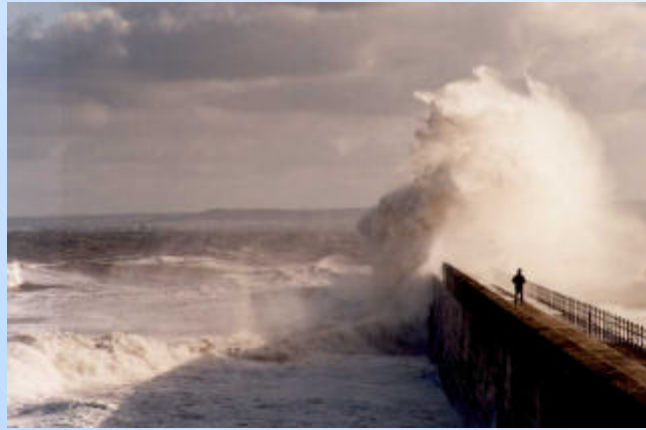
Figure 1: Heugh Breakwater, Hartlepool, UK (Photo courtesy George Motyka, HR Wallingford)
